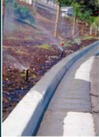
Not all water applied to landscapes is used by plants. Some is lost due to runoff, windspray, or deep percolation. Irrigation efficiency losses need to be included in water budget calculations.
